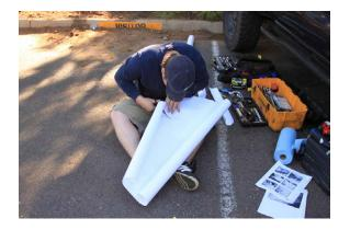
Secure the template on to the truck's body, using the body lines to matchup with the template. Using a center punch, mark where indicated on the template. These holes will be the mounting points of the snorkel as well as the hole used for the intake coming from the snorkel into the fender. When all hole centers are marked, remove the template and make sure you are up to date on your liquid courage.
